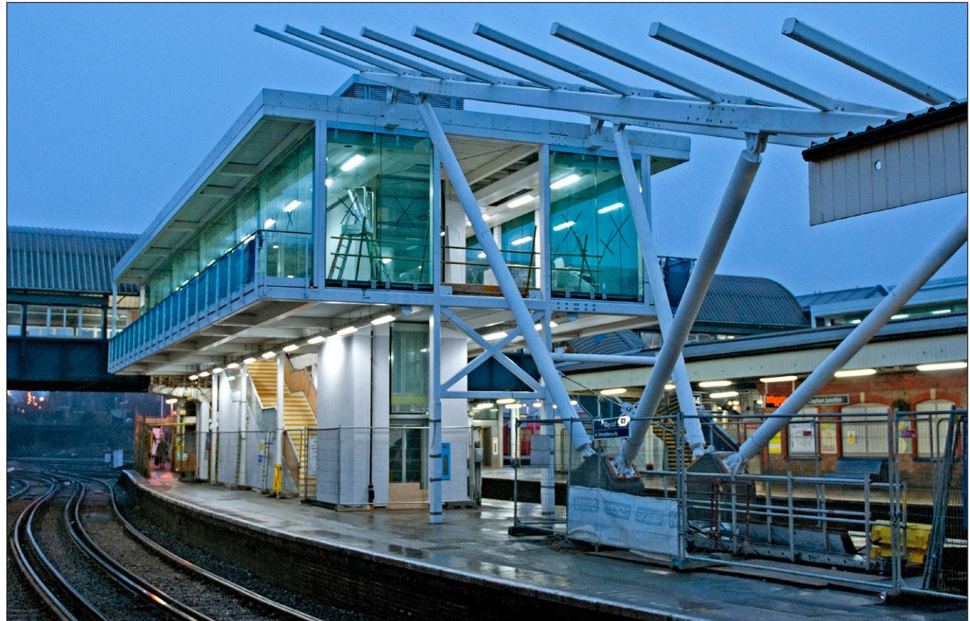
▲ Except for Platform 17, from where this view was taken, all platforms at Clapham Junction now have lifts installed. In addition Platforms 13-16 are being provided with this design of covered walkway and lift. Bill Turvill
